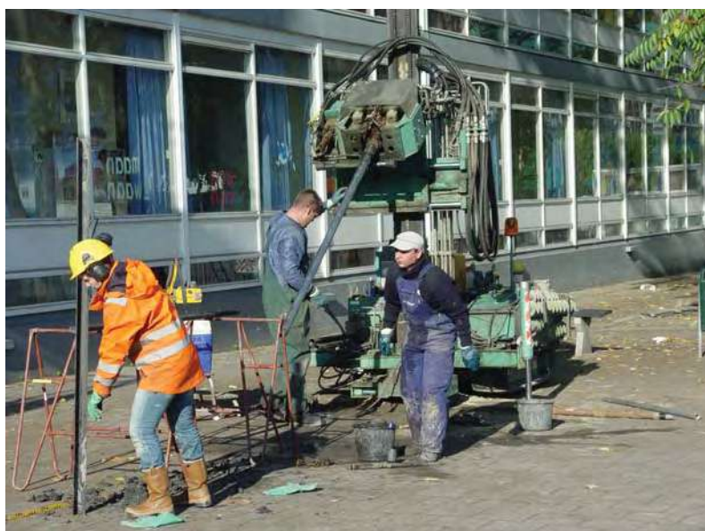
Figure 13.3: Mechanical borehole surveying at the Rotterdam Markthal site. Photo BOOR.
