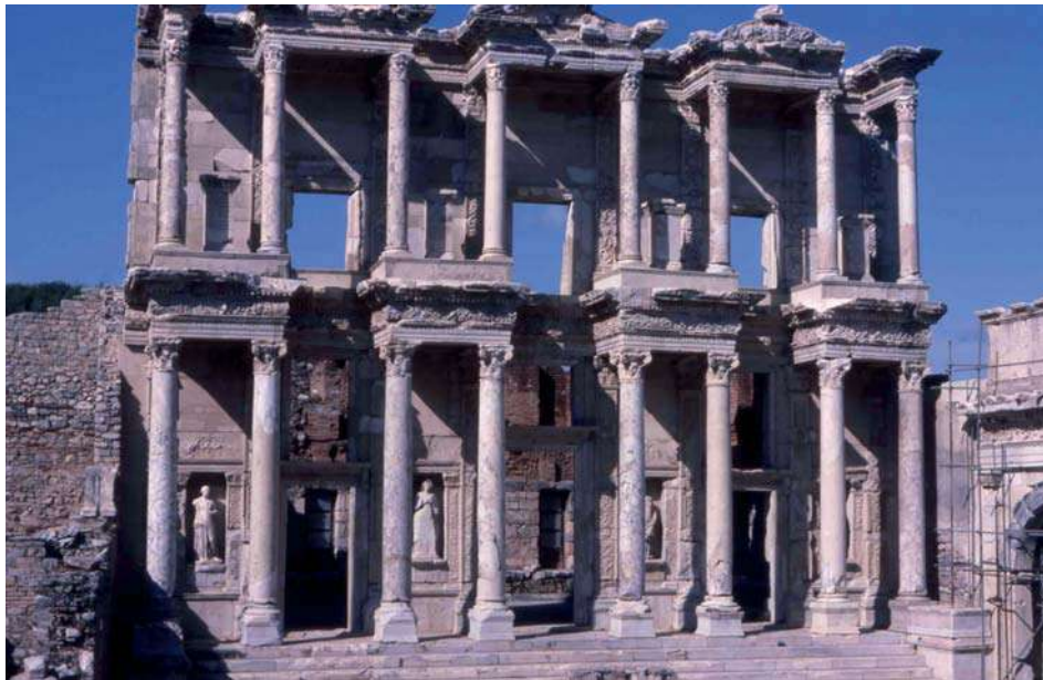
Figure 4. The facade of Celsus Library in Ephesus was erected in the 1970s with anastylosis technique. (Photo: 1990, Mehmet Özdoğan)
