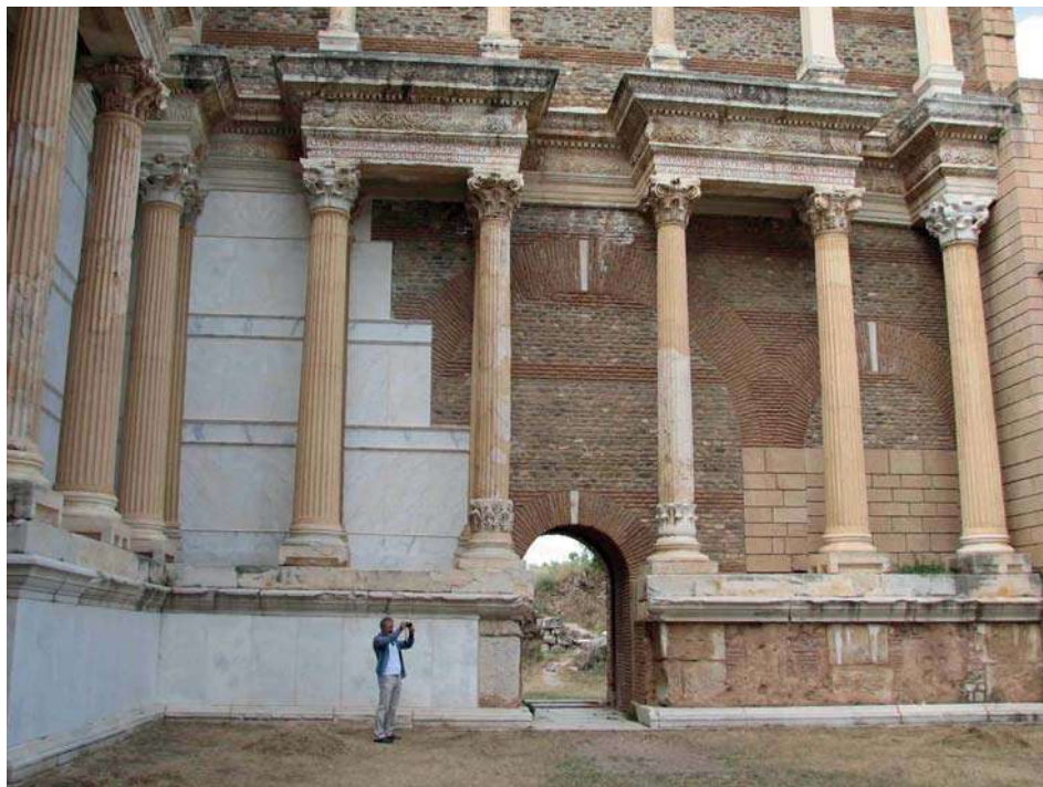
Figure 6. A detail from Sardes Gymnasium; most of the masonry and marble coverings were made with new material. (Photo: 2013, Zeynep Eres)
