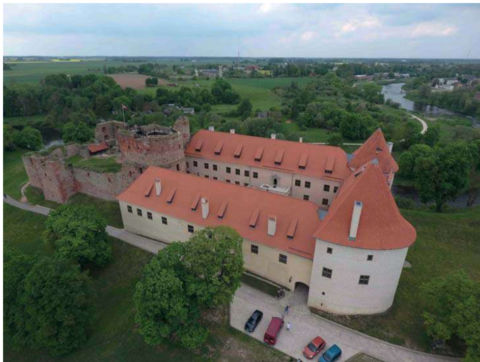
Figure 1. Bauska Castle complex consists of a medieval fortress built in the middle of the 15th century and a ducal palace constructed in the mannerist style in the late 16th century. (Photo: E. Šulcs)
