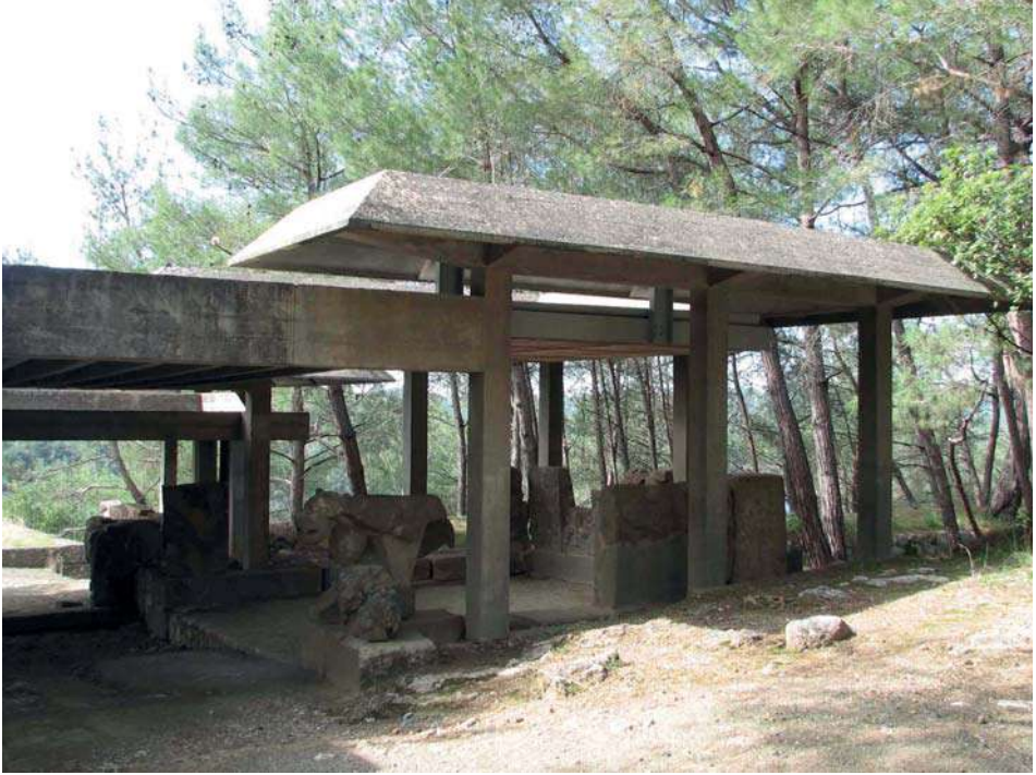
Figure 3. The roof was built between 1957–1961 to protect the Karatepe-Aslantaş orthostats in situ . (Photo: 2015, Zeynep Eres)
