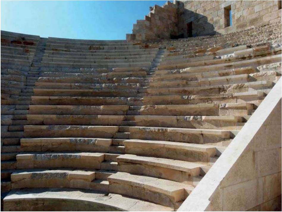
Figure 17. A detail from the bouleuterion in Patara ancient city. All the stairs were reintegrated with new material for using the building for social activities and unfortunately, the authenticity of the building is totally lost. (Photo: 2015, Merve Arslan Çinko)
