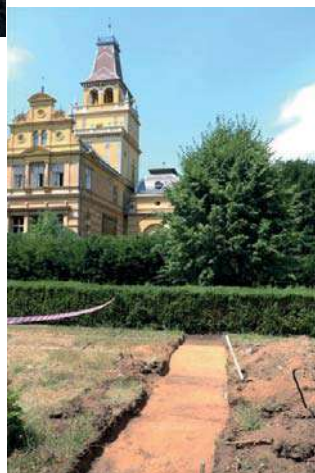
Figure 17. Foundation of the pathway in front of the mansion's southern facade
