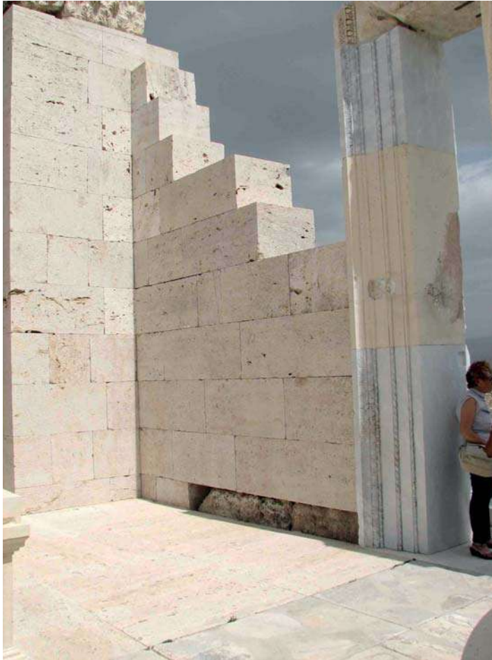
Figure 16. A detail from the temple implementation in Laodicea: A single row of original stone is visible on the ground, the upper part of the wall was built completely with new stones. (Photo: 2013, Zeynep Eres)
