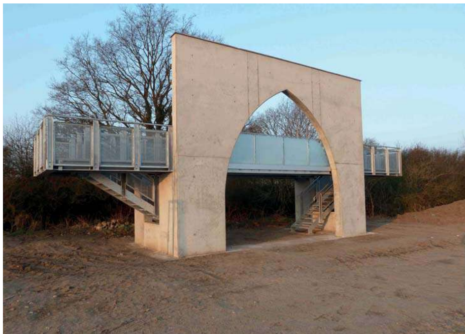
Figure 15. The new town gate with its view point platform (C. Krauskopf, BLDAM)
