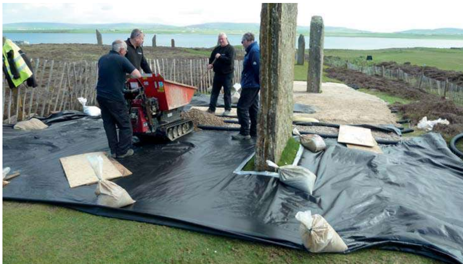
Figure 14. Installation of new raised path to part of the inner ring route, 2017. © Historic Environment Scotland
