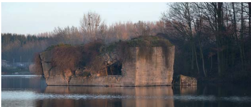
Demolished bunker of the so-called Westwall in a flooded gravel pit near Hückelhoven. (W. Wegener, LVR-State Service for Archaeological Heritage)
