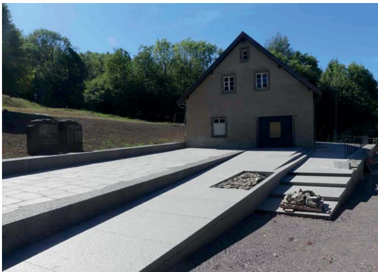
Figure 3. KL Natzweiler-Struthof, Natzwiller, Bas-Rhin, Communauté européenne d'Alsace. The new memorial of the gas chamber, built after the archaeological surveys, summer 2022 (© V. Carpentier, INRAP)
