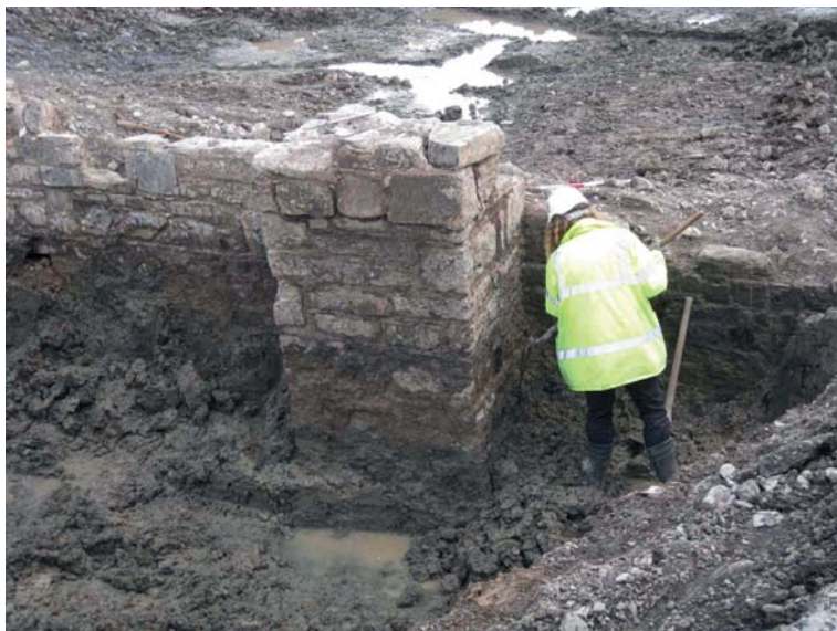
Figure 3. Cleaning newly exposed buttresses and retaining walls, Broadstone Harbour
