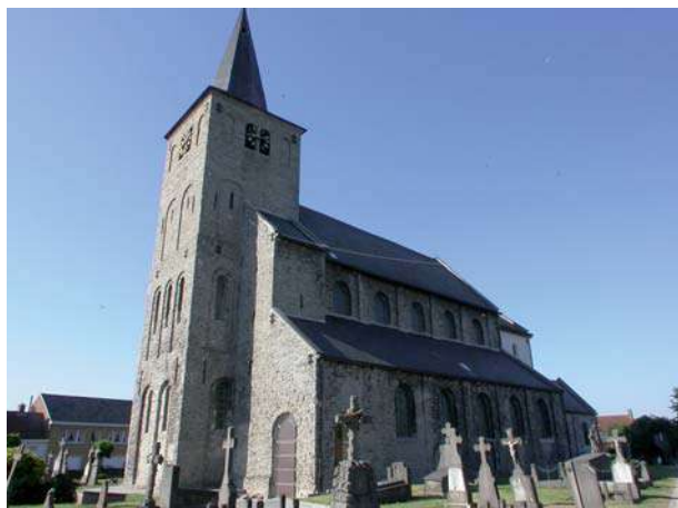
Fig. 21.2: Ename. The present Saint Laurentius church has preserved its original architecture to an important extent (Daniel Pletinckx - Visual Dimension bvba).
