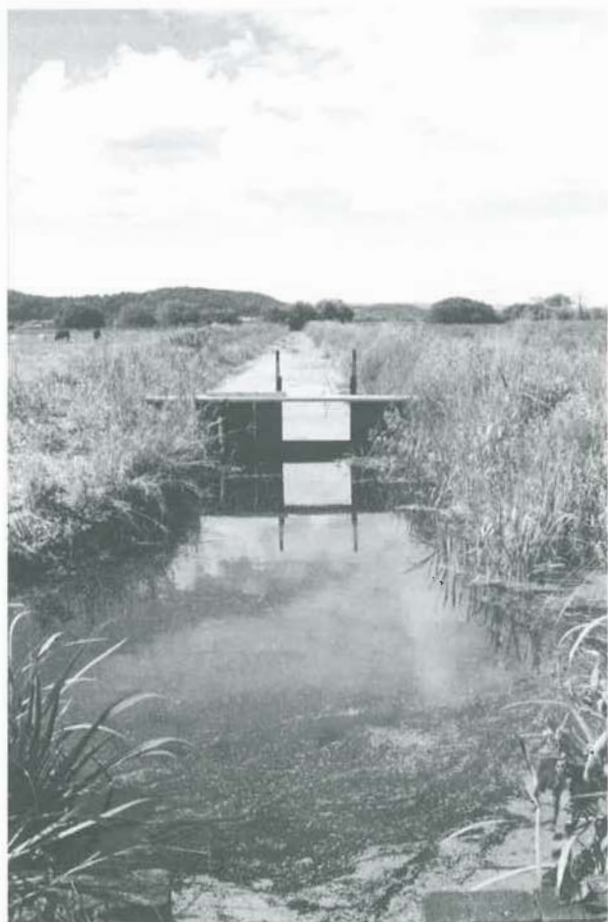
Fig. 4.6: A stop log sluice on the West Sedgemoor RSPB reserve, Somerset, used to control the ground water level of the reserve. Note the grazing cattle, an important part of the reserve's management system.
