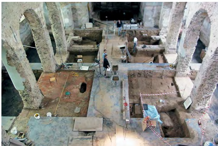
Fig. 7.7: Excavations in the nave of the Saint Laurentius church.
