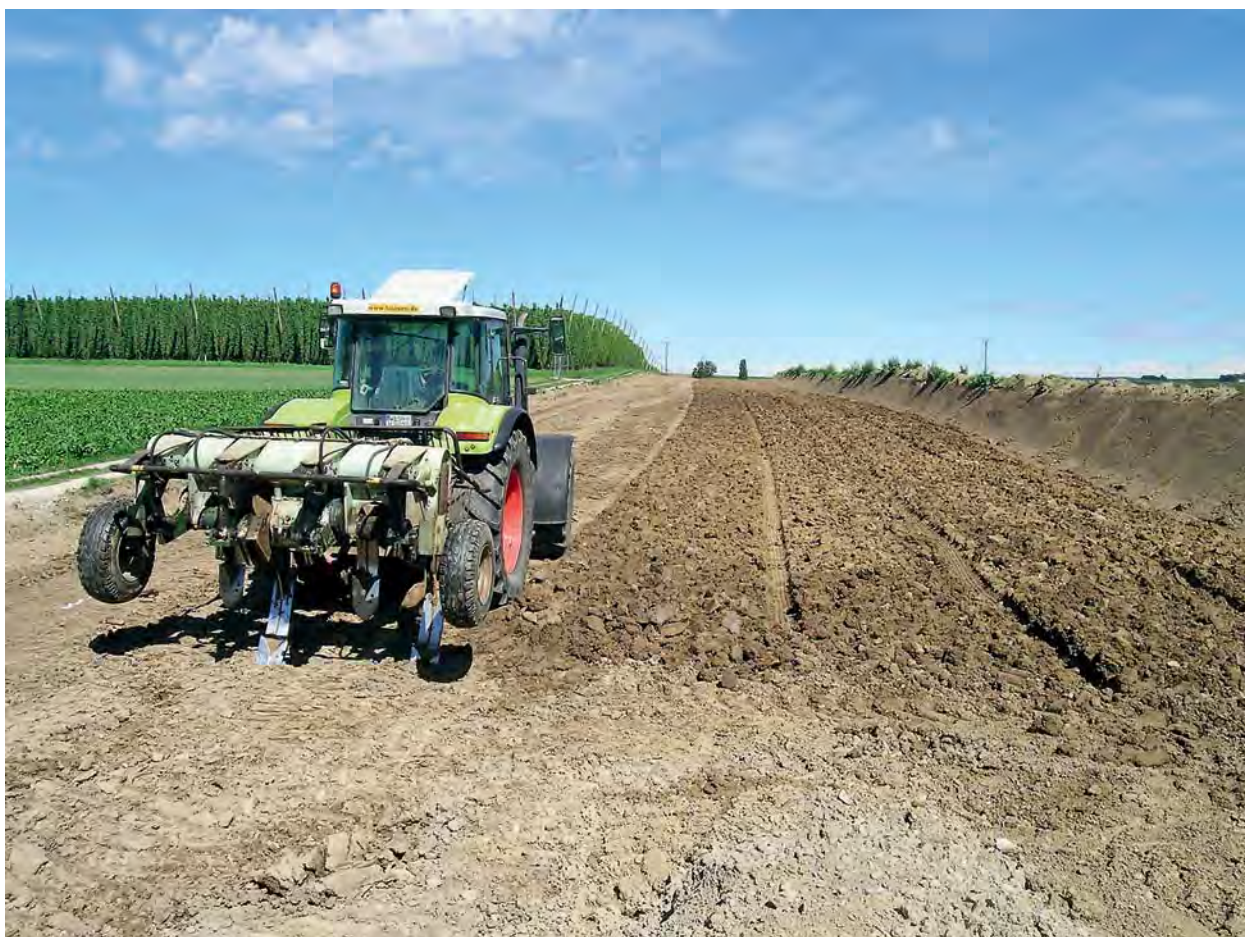
Fig. 13.8: After refilling the pipe trench, the surface is flattened and deep-ploughed (gas pipeline Irsching–Forchheim, Lkr. Eichstätt).
