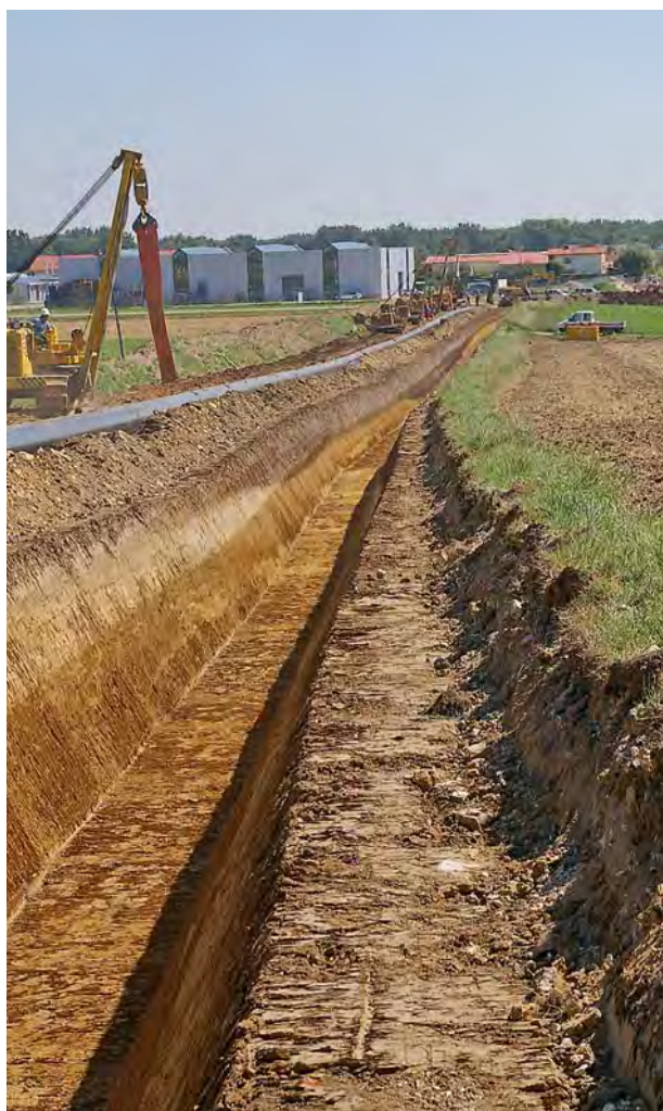
Fig. 13.6: The route of a gas pipeline 500 m east of the Roman fort Celeusum (Pförring, Lkr. Eichstätt, Reg.-Bez. Oberbayern) showing the pipe trench after finishing the excavation. A Roman ditch is visible under the colluvial covering that protected the surviving archaeological features.
