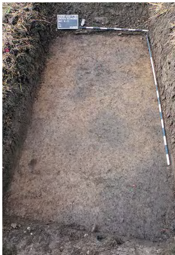
Fig. 13.8: After refilling the pipe trench, the surface is flattened and deep-ploughed (gas pipeline Irsching–Forchheim, Lkr. Eichstätt).
