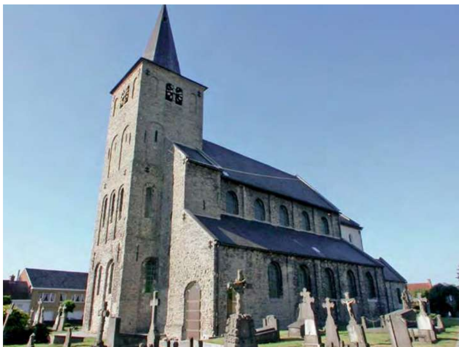
Fig. 7.12: Ename, Saint Laurentius church. View from the northeast of the restored church with its eastern part richly decorated with blind arches.
