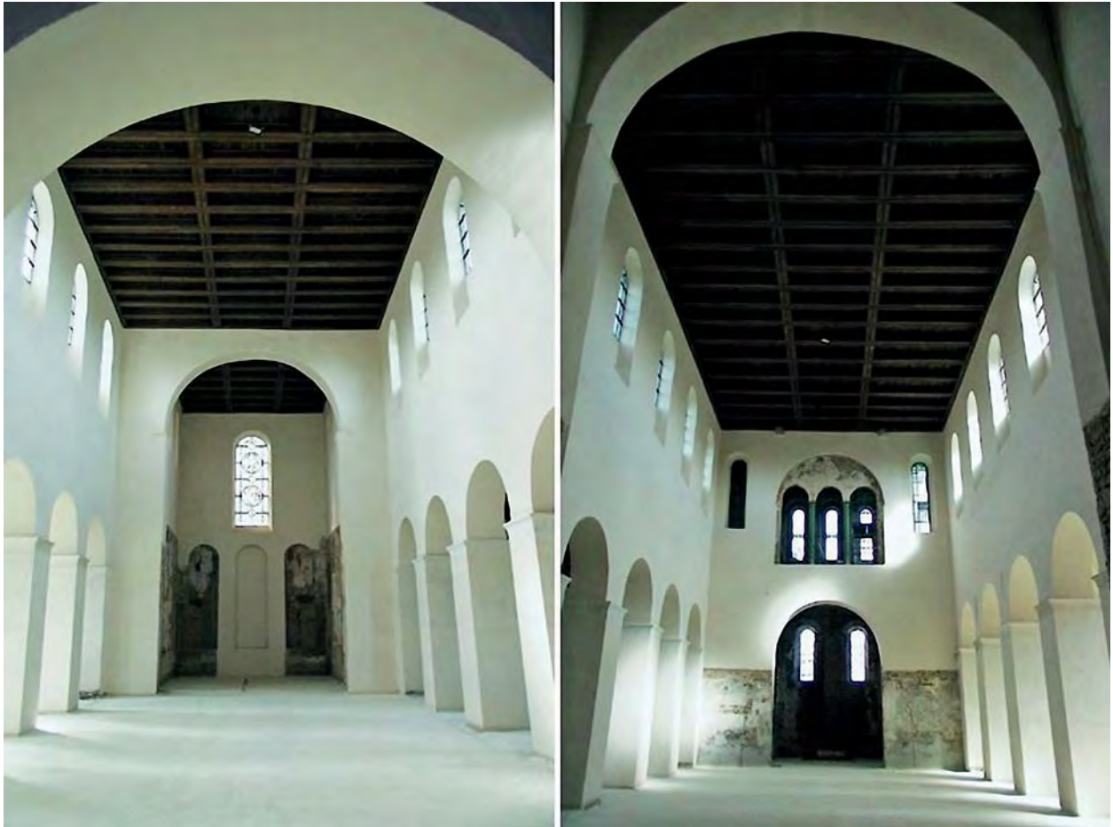
Fig. 7.16: Ename, Saint Laurentius church. The central axis after the restoration. Striking elements of the east choir (right) are the two altar floors and the triple arcade on the second level with the mural of the Majestas Domini on top.
