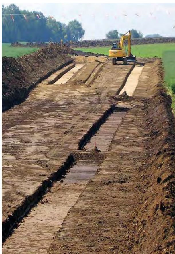
Fig. 13.7: Removing about 0.30–0.40 m of the topsoil with a wide-shovelled excavator brings good results. With a second excavator the remaining surface is cleared away either in stripes or laminar under the supervision of an experienced member of the excavation team (gas pipeline Irsching–Forchheim, Lkr. Eichstätt).
